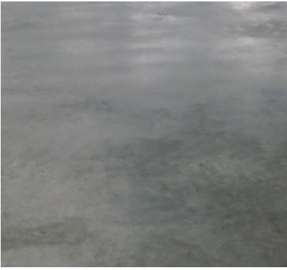
Power floated screed
